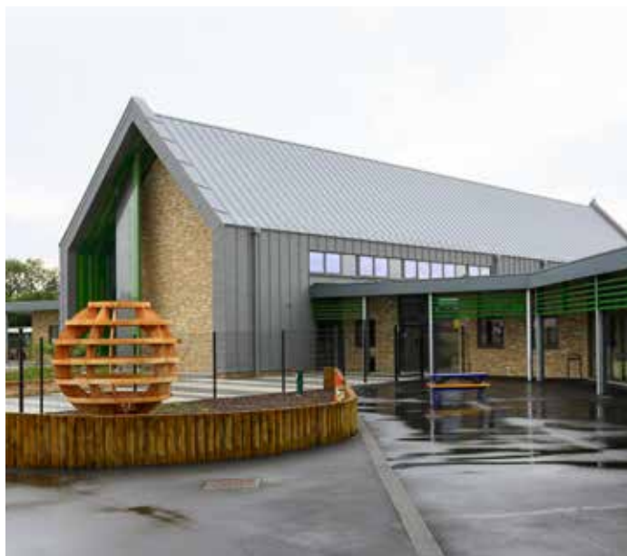
Rosecroft Primary School, Norfolk (UK) - Architecte : NPS (South East) Property Consultants - Entreprise : ZINK.IT
